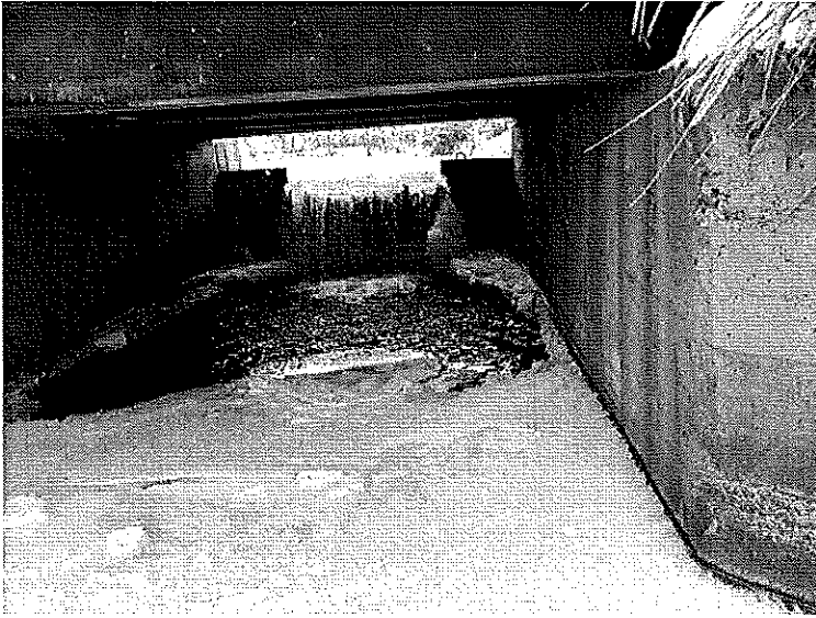
Photograph 1 Looking upstream at the existing diversion structure.
